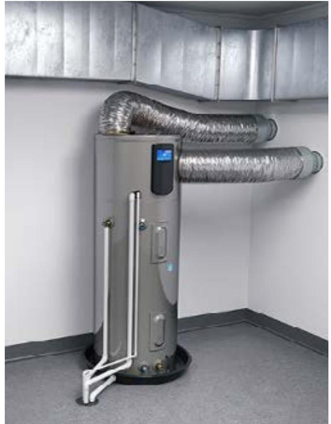
*Heat pump water heater ductwork for air intake and exhaust*
